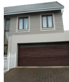
Typical Garage Door
