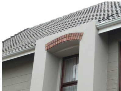
Red Face Brick Plinths
