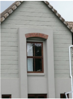
Typical External Wall finish to Second Level
